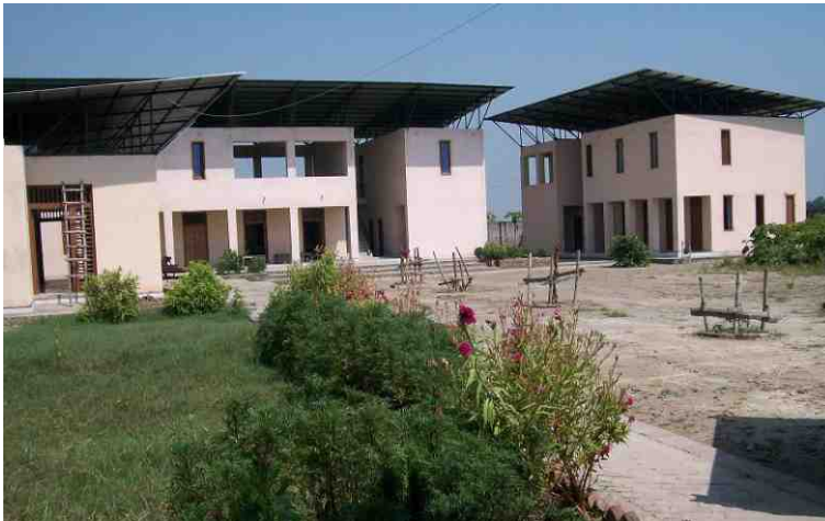
Rehabilitation centre for girls under construction in Faizabad
